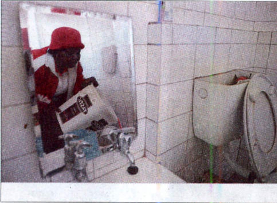
Leah Thelele, a resident of a Joburg council-owned block of flats in Windsor East, has to find ways to flush her toilet. She has been without water or electricity for almost two years. PICTURE: MUJAHID SAFODIEN
